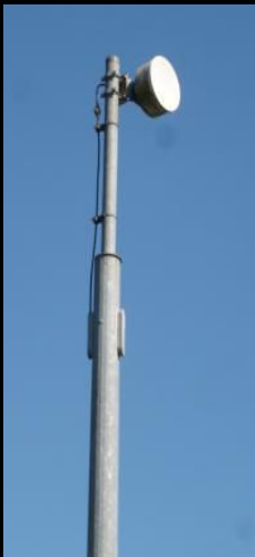
The exchange has a microwave link to the Canterbury exchange.
