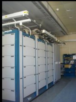
There is a window with a nice view of the comms racks....
