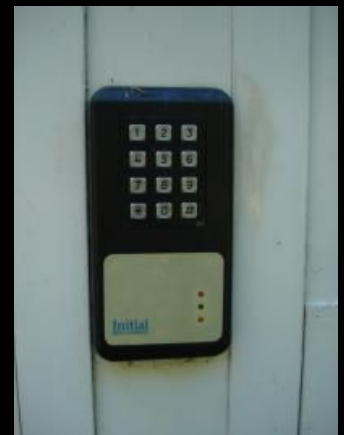
So, they've disconnected these, then? (so why are the lights still on?)
